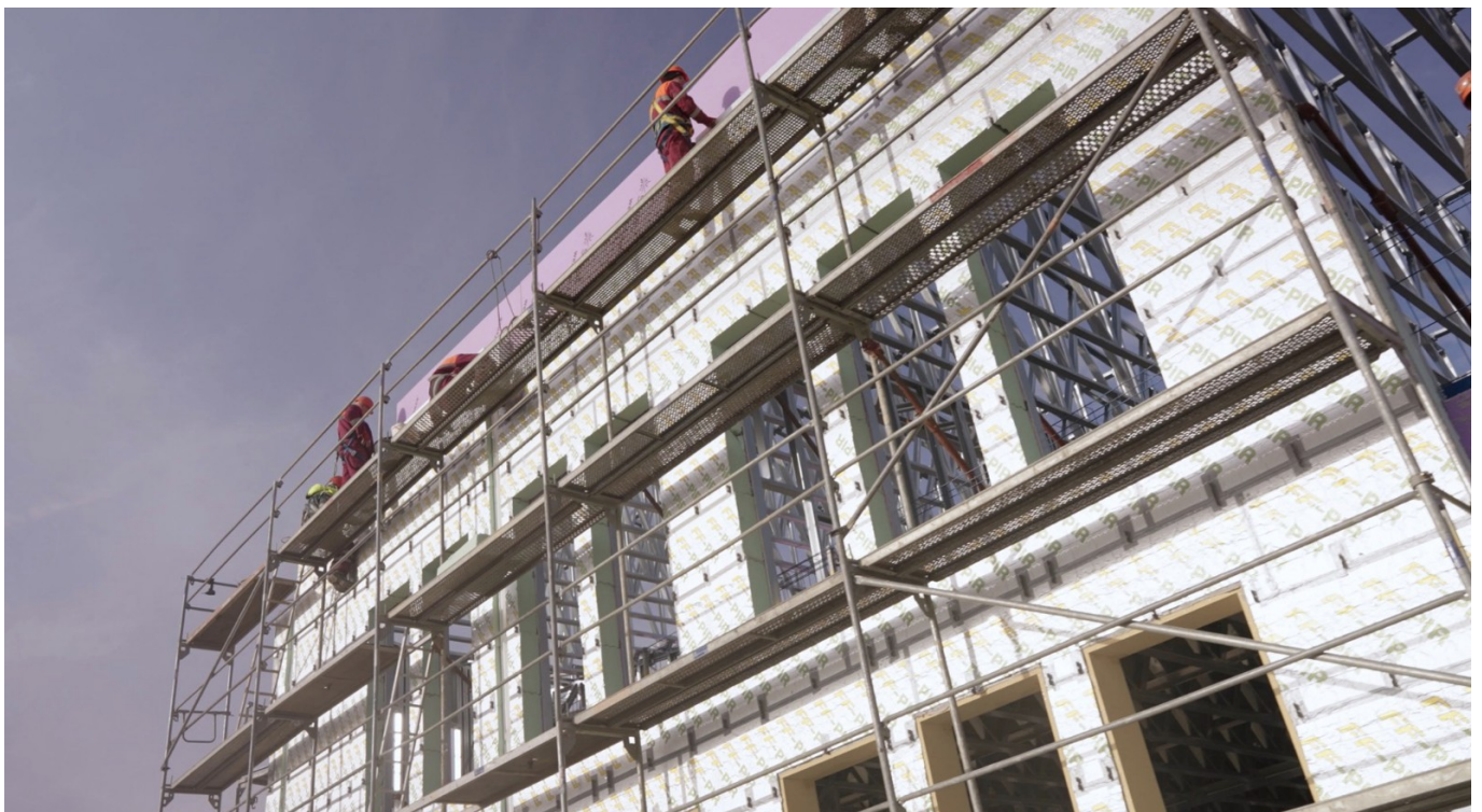
REAL NP5 PROJECT / CONSTRUCTION STAGE
