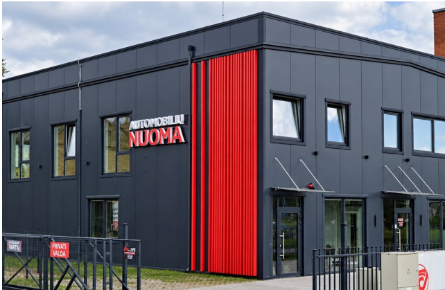
BUILDING ON SITE
